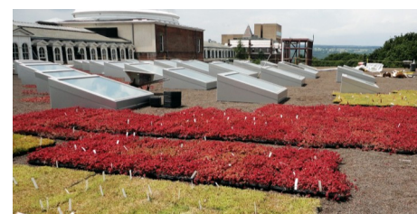
The roof has been planted with two different species of Sedum, as specified by the architect.
