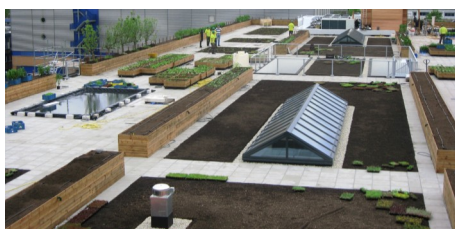
The system build-up "Sedum Carpet" with Fixodrain® XD 20 was applied between the skylights ...
