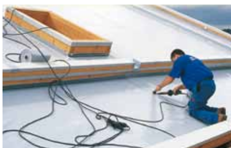
The roof area to be greened is sealed with rolls of waterproofing membrane that have been tested for their root-resistance (in line with FLL procedures.)
