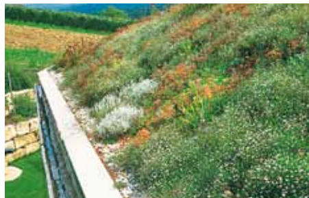
Even after only one vegetation period the plant coverage is largely complete. The roof area in this example is drained by means of an outer-lying gutter into which the three water spouts carry any excess water.
