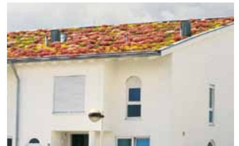
A shear barrier is placed just above the eaves on this monopitch roof, which is drained by means of an outer-lying gutter.
