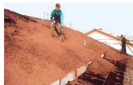
Depending on the roof pitch, growing media Zincoblend E or Zincoblend I is applied onto the roof until the Georaster® elements are filled and covered up to a total depth of about 4.25 in.
