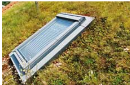
This roof with a pitch of approx. 1/12 is drained using a gutter and does not yet require any special measures.
