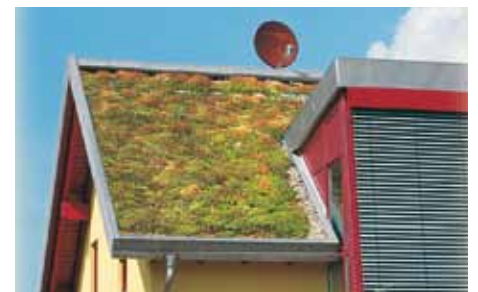
With this roof, which has a pitch of approx. 7/12, a shear barrier was installed within the roof area, in addition to the stable eaves.
