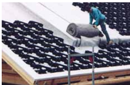
Once the area has been covered with the Protection Mat WSM 150, the Georaster® elements are installed, starting from the bottom up.
