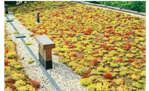
This roof with a pitch of approx. 1/12 is drained using a gutter and does not yet require any special measures.
