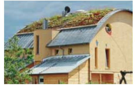
Sometimes it is a matter of structural design, as can be seen here (extreme pitch in the lower roof area), that leads to two different "coverings" being used on the same building.
