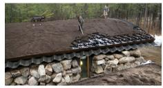
In the next step the drainage elements were completely filled with the growing media.
