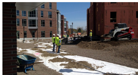
The System Filter Sheet PV has been installed below and on top of Stabilodrain® SD 30.
