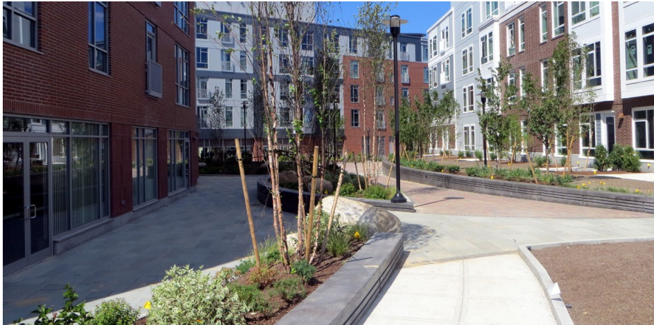
This photograph hardly reveals that this beautifully designed courtyard is located on a roof.
