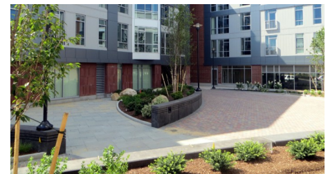
The planting areas have been separated from the hardscape areas by low curbs on one side and by benches on the other side.
