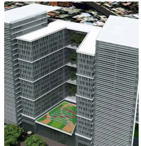
The first building of the new district "Nueva Las Condes" in Santiago de Chile provided with a green roof.
