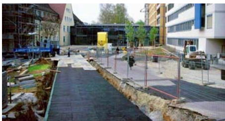
Installation of the Elastodrain® EL 202 under the hospital driveway.
