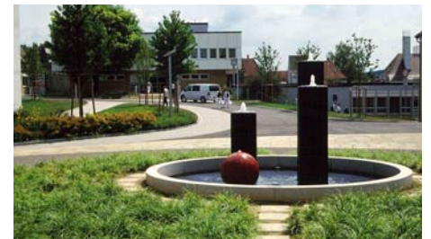
Planting beds, a water feature as well as walkways and driveways were installed on top of the hospital's basement.
