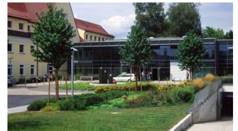
A small park was created in front of the main entrance to the hospital.
