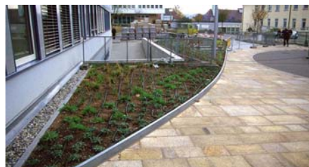
On the substrate surface the water hoses of the drip irrigation can be seen.
