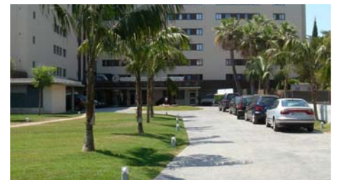
The same view after completion.
