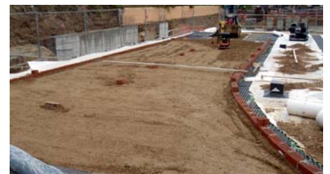
Applying the base layer.
