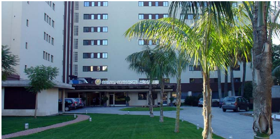
Hotel access for minibuses and cars on top of a two story deep underground garage.
