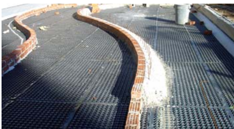
Curb between driveway and green zone.
