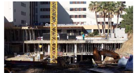
The underground garage under construction.
