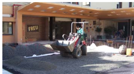
Application of gravel with a wheel loader.
