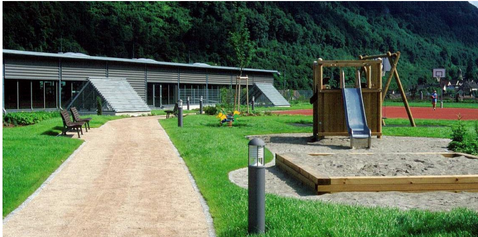
The main roof area after completion in July 2002.
