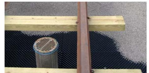
Installation of the green roof build-up under the rails. The drainage layer consists of infilled Floradrain® elements.
