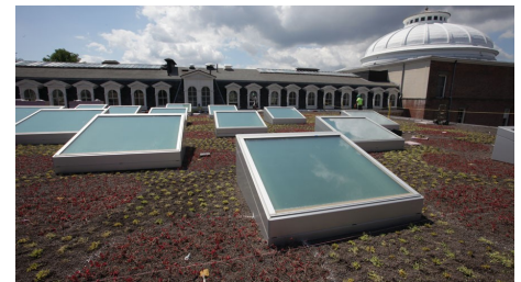
The numerous skylights provide the rooms below with sufficient light.
