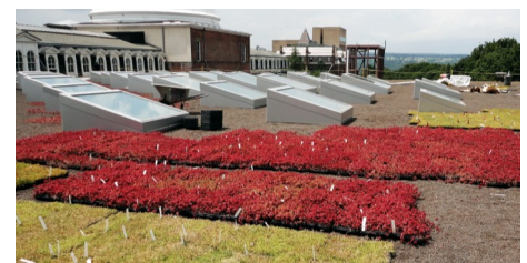
The roof has been planted with two different species of Sedum, as specified by the architect.
