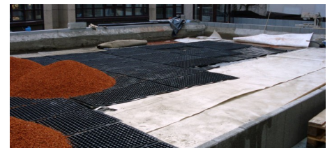
Installation of the Stabilodrain® SD 30 elements in an inner courtyard.
