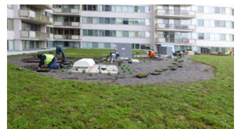
Most of the roof area was planted with pre-cultivated plant mats to achieve an immediate green effect. In the area around the technical installations different higher-growing grasses were planted.
