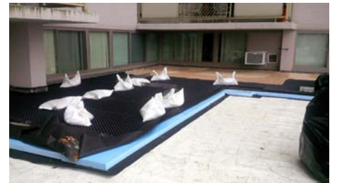
The roof of the building was built as an inverted roof.
