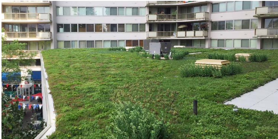
Besides the reduction of water runoff, the green roof also enhances the visual appearance of the surface.
