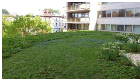
Most of the roof area was planted with pre-cultivated plant mats to achieve an immediate green effect. In the area around the technical installations different higher-growing grasses were planted.
