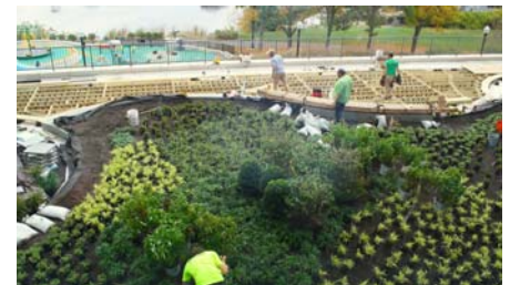
Floradrain® FD 40-E is the core element of the vegetated areas providing the plants with an optimal water-/air balance.
