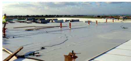
Preliminary work on the roof area to be vegetated.
