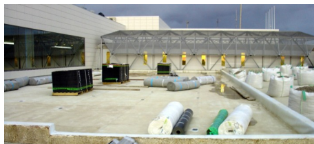
Protection mat, drainage elements and filter sheet are ready for installation.
