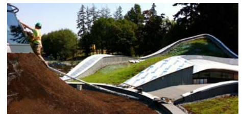
Shortly before completion of the roof surfaces.
