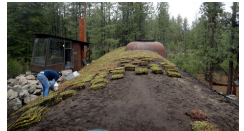
In order to obtain a complete green coverage immediately pre-cultivated vegetation mats have been applied on the growing media.
