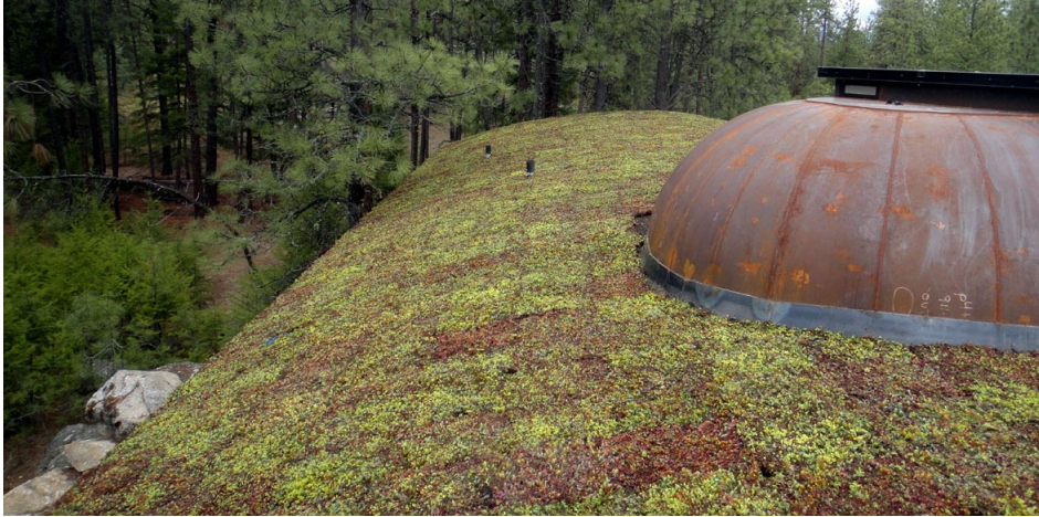
The green roof integrates the building perfectly into its surroundings.
