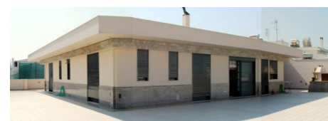
The terrace before reconstruction...
