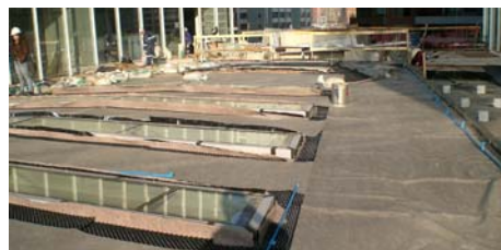
The irrigation pipes were installed above the filter sheet, the entire surface beneath is covered with Floradrain® elements.
