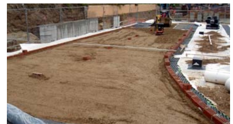
Applying the base layer.
