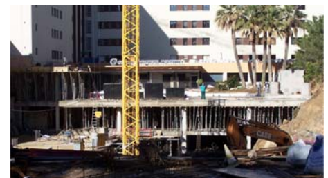
The underground garage under construction.
