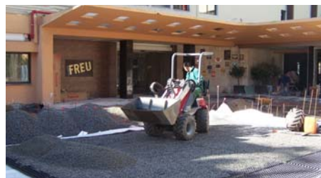
Application of gravel with a wheel loader.
