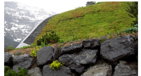
The sloped roof with newly-installed pre-cultivated vegetation mats.
