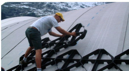
The Georaster® elements are installed from the bottom up. In the background, the legendary Eiger North Face.
