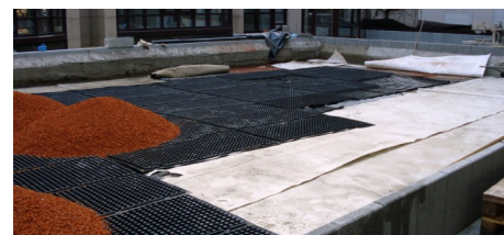
Installation of the Stabilodrain® SD 30 elements in an inner courtyard.
