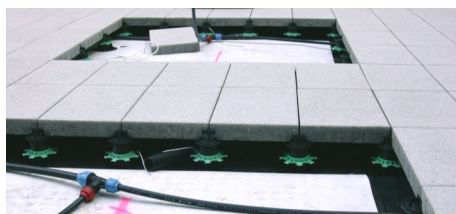
Under the elevated concrete slabs was enough space for the irrigation pipes.
