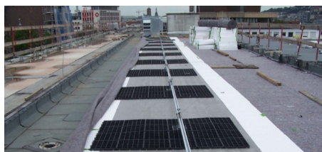
The ZinCo ballast held fall protection system was installed on the upper green roof area.
