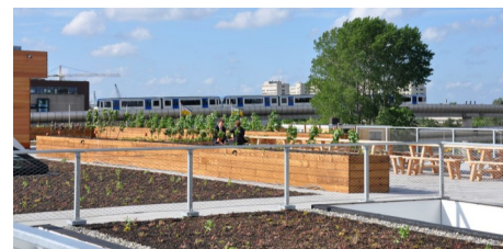
In the foreground: The areas with extensive green roof vegetation shortly after completion .
