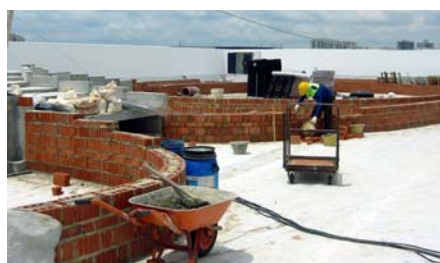
Features such as ramps and bridges were built on top of the protection and drainage layer.
