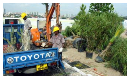
Local palm trees were planted in a 1,20 m deep substrate layer.
