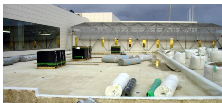
Protection mat, drainage elements and filter sheet are ready for installation.
