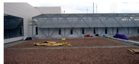
The roof area just after the application of substrate with Big Bags.
