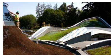
Shortly before completion of the roof surfaces.
