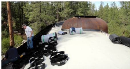
In the steeper areas the Georaster®-elements have been placed on the Water Retention Mat WSM 150, starting from below.
