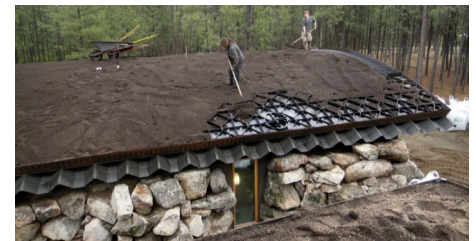
In the next step the drainage elements were completely filled with the growing media.
