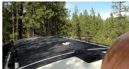
In the flatter areas above the Georaster®-elements Floradrain® FD 40-R have been installed.
